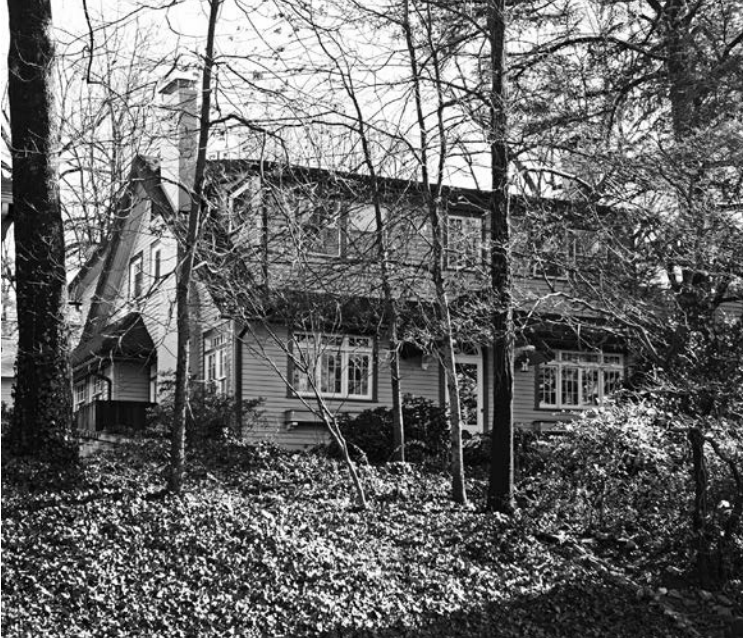
The 1911 Follin House in West End, 1232 Glade Street. Photo by Jackson Smith, 2019
